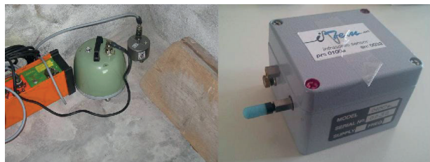
Fig. 2 – Seismic (left) and infrasound (right) sensors installed in Fadalto.
