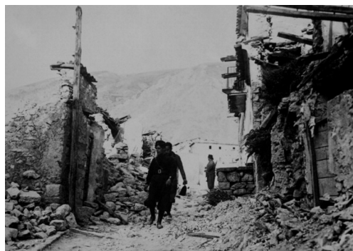
Fig. 1 – View of the severe damages in one of the villages east of the Maiella massif (photo Keystone-France/Abruzzes/gettyimages).
