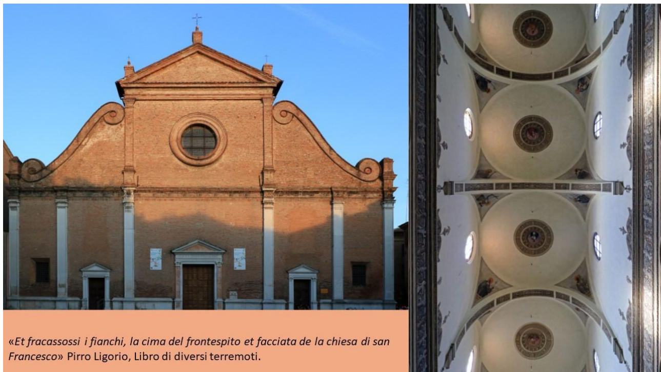
Fig. 3 – The upper portion of San Francesco, above the frame of the order, and the internal domes and circular windows rebuilt after the 1570 earthquakes. Italian quotation from Pirro Ligorio's writings, describing the collapse.
