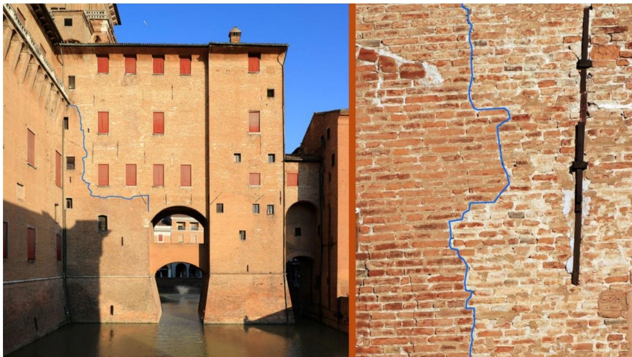
Fig. 2 – The hasty reconstruction of the ducal apartment over the Estense Castle southern barbican, using recycled bricks and limestone fragments, following the large collapse of November 17, 1570.
