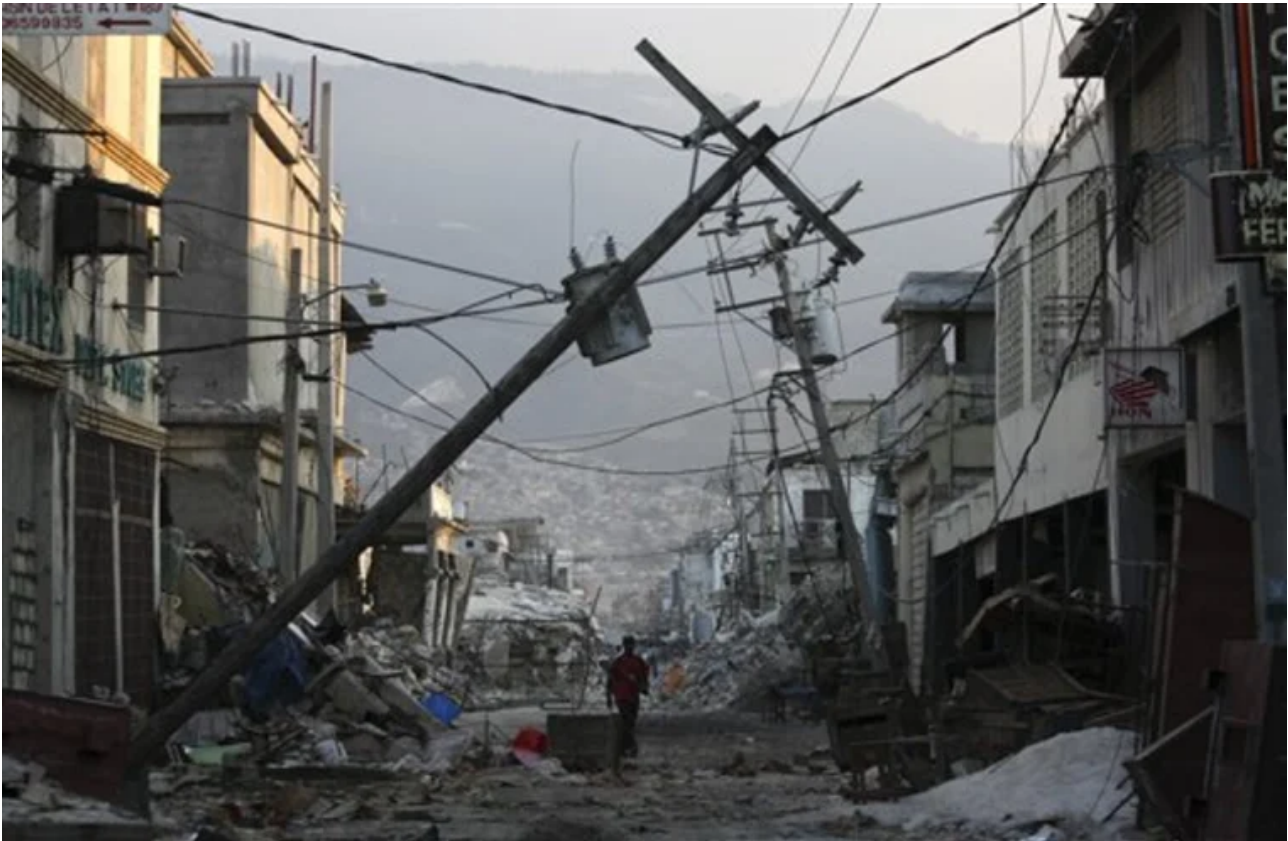
Fig. 3 – Photo taken February 16, 2010, a man walks down an earthquake damaged street with fallen electrical lines in downtown Port-au-Prince; source: The Associated Press
