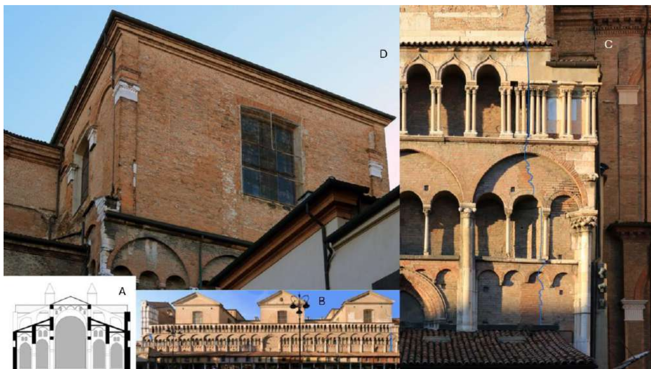
Fig. 1 – A reconstructive cross section of the Ferrara Cathedral after the 13 th century post-seismic restoration (drawing by A. Toma and V. Vona), B southern side of the Cathedral, with the main structural lesions induced by foundation settlement and seismic acceleration depicted in blue, C the south-eastern corner, with post-seismic collapse transept reconstruction in a backward position and “wall sewing up restoration” by reddish bricks, D the Renaissance transept rebuilt at the end of the 15 th century and partially collapsed during the earthquake of 17 Novembre 1570.
