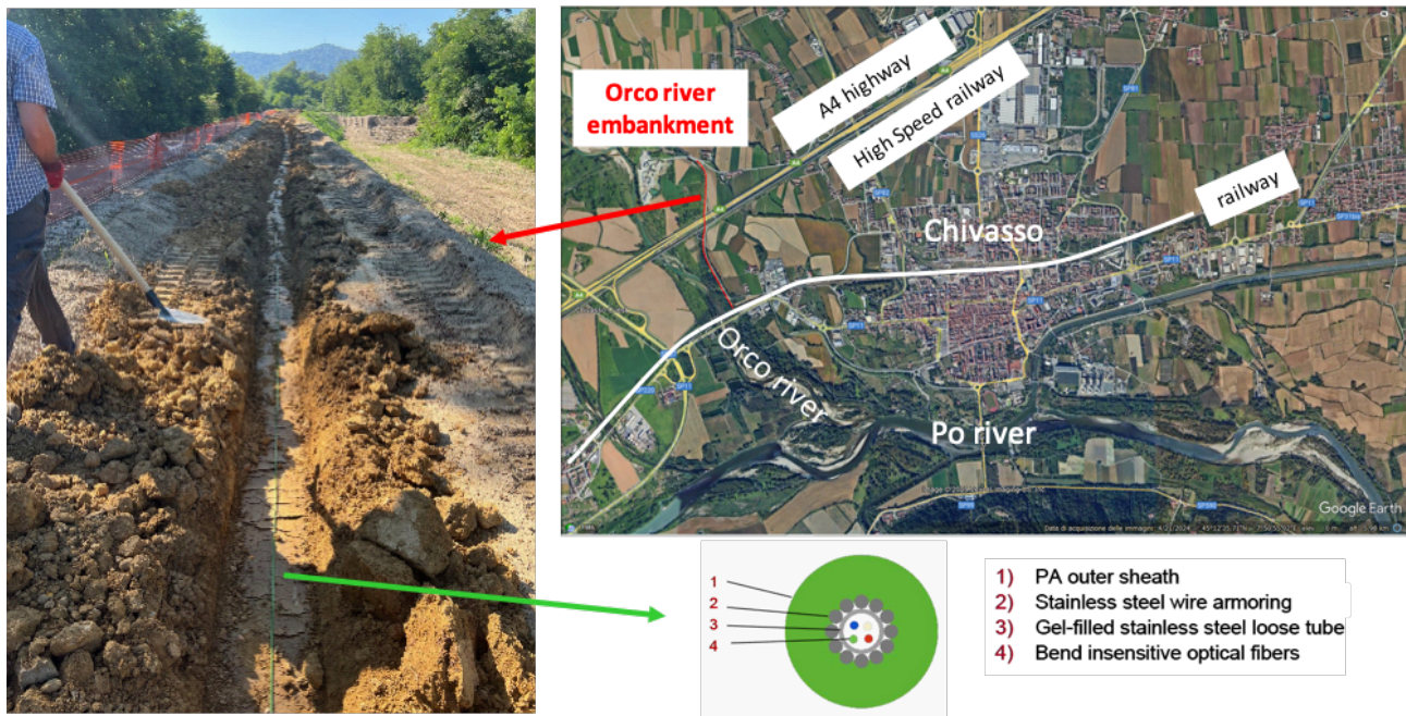
Figure 1 – Location of the test site and of the DAS cable installed over the embankment.
